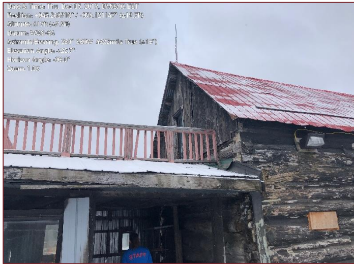
Site Photograph 1 – Barn Exterior
