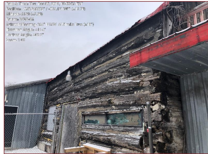
Site Photograph 2 – Barn Exterior
