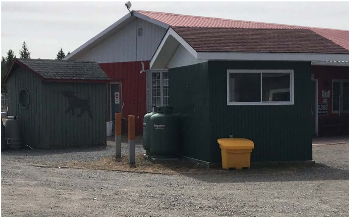
Kennel building with two sheds in foreground
