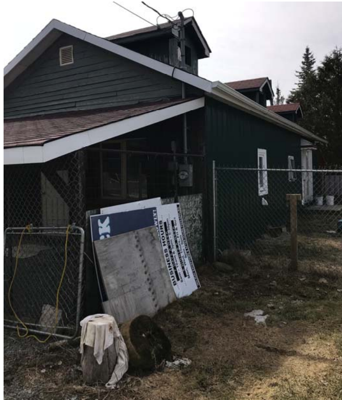
Shop building (laundry and tool shed)
