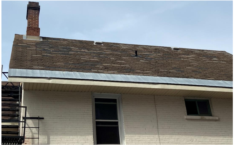
11 Roof and chimney of 230 Lisgar. MTBA
