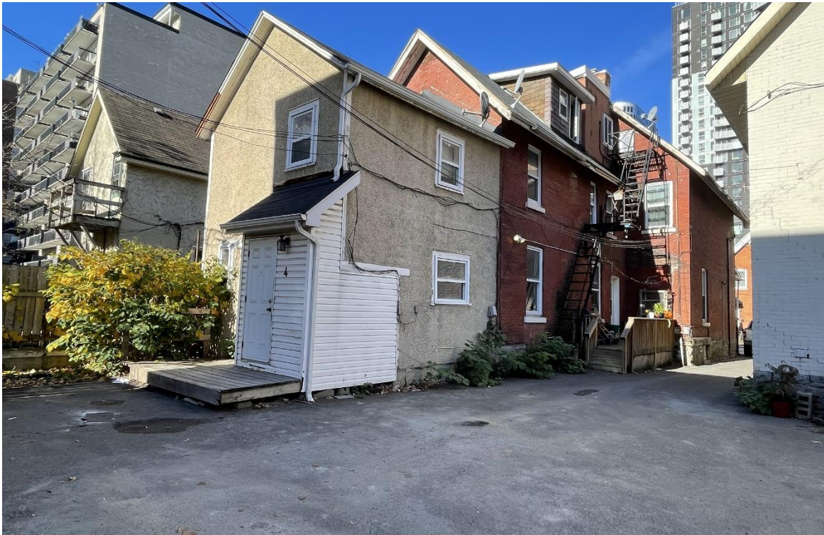
Photograph 3: View of the 232 Lisgar Street, looking northwest.
