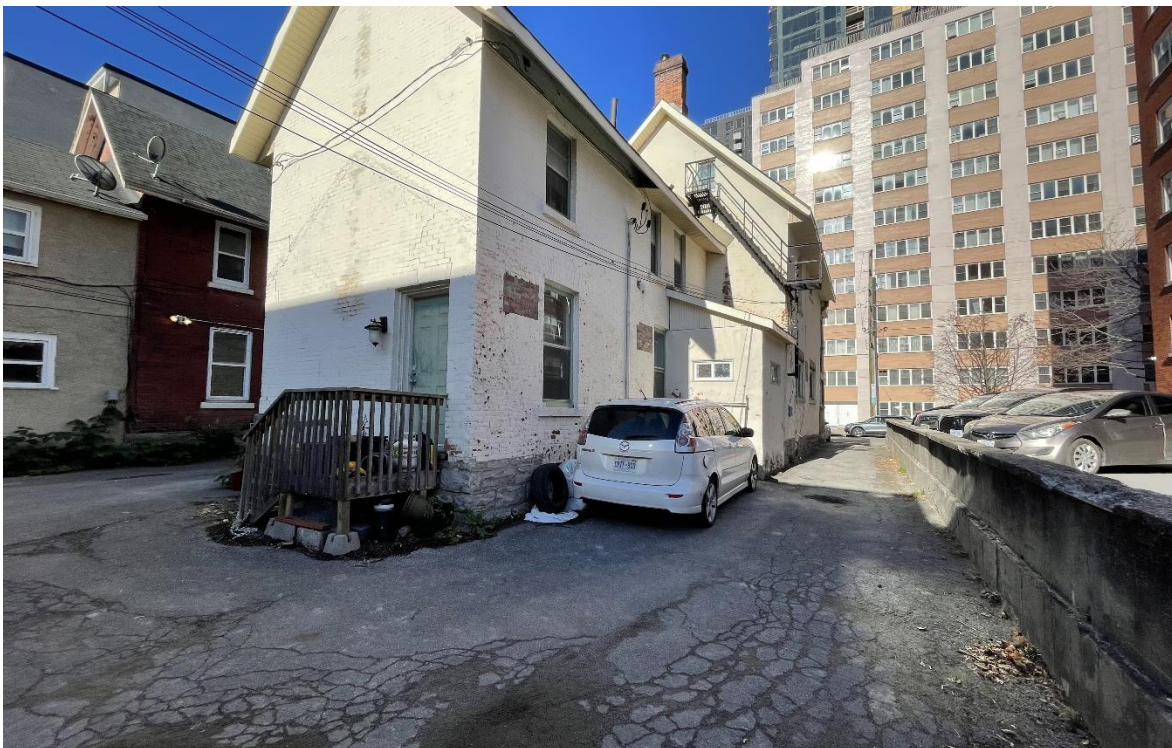
Photograph 4: View of the 230 Lisgar Street, looking northwest
