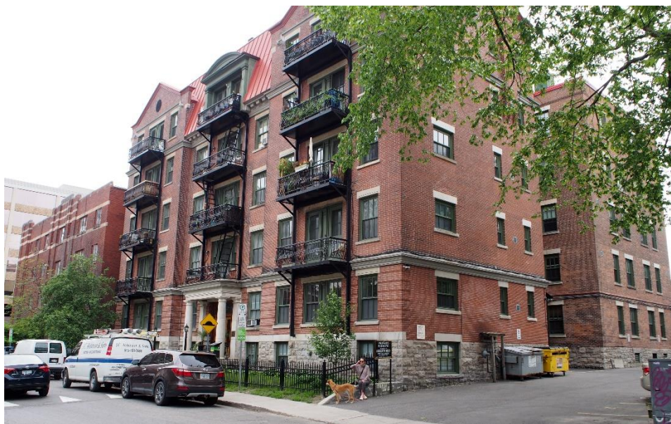
45 The Shefford, designated under Part IV of the Ontario Heritage Act. MTBA
