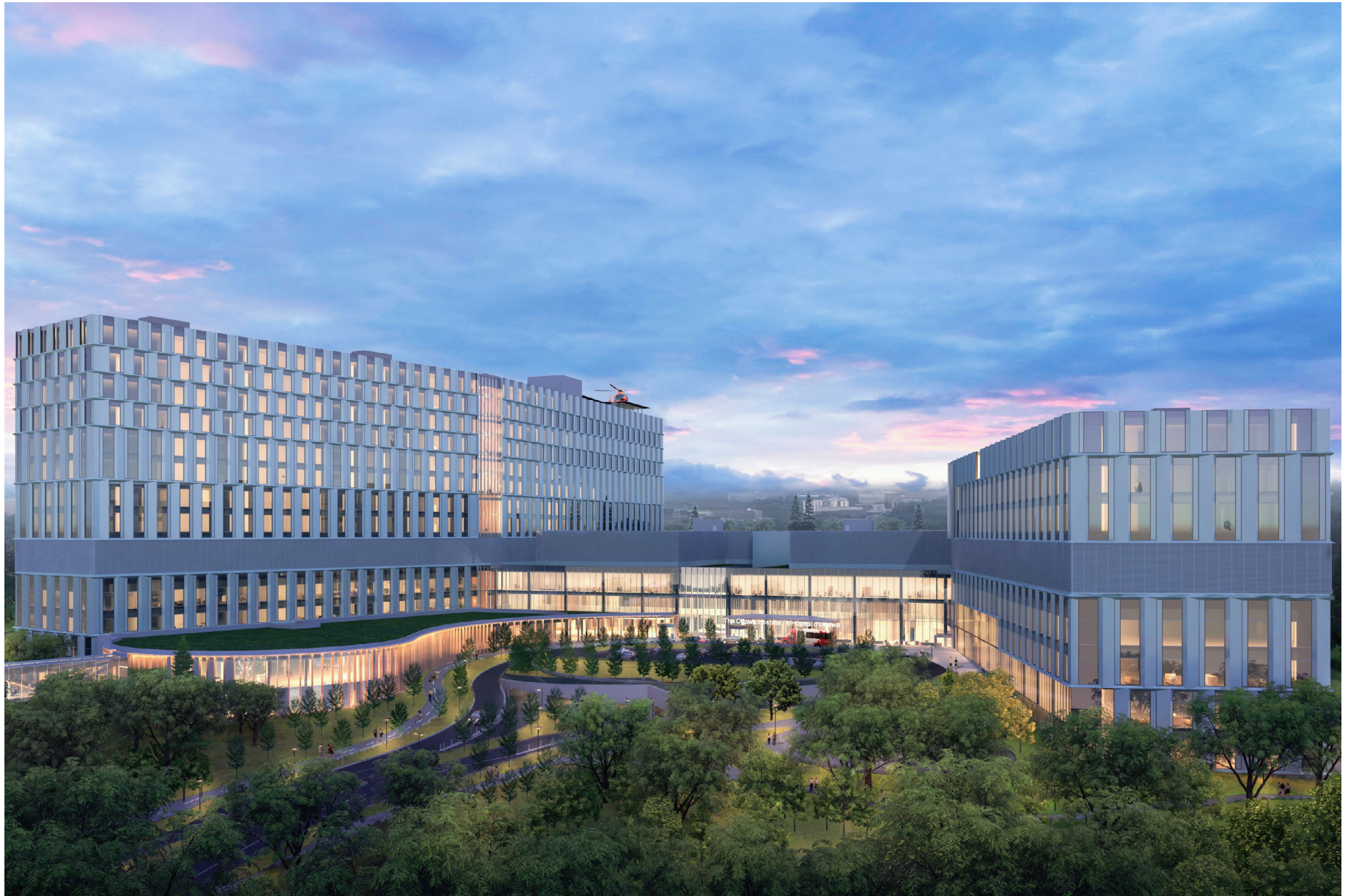
Figure 77: Hospital Main Plaza - Evening
