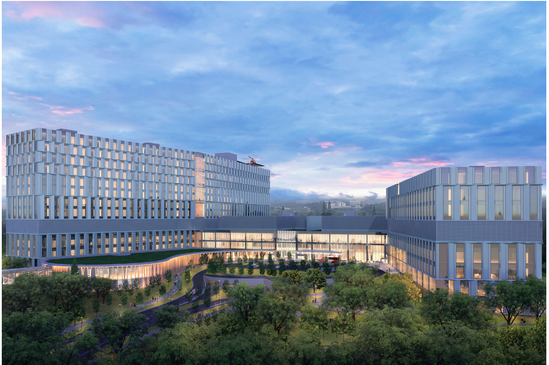
Figure 78: Hospital Main Plaza - Evening
