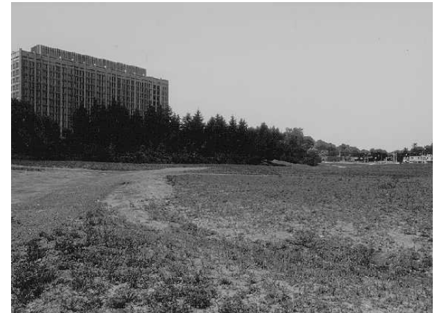
Figure 72: The Original Sir John Carling Building, viewed from the northeast towering over the escarpment
