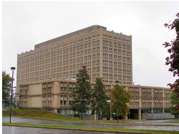
Figure 71:The Original Sir John Carling Building, viewed from the southeast making use of the natural topography
