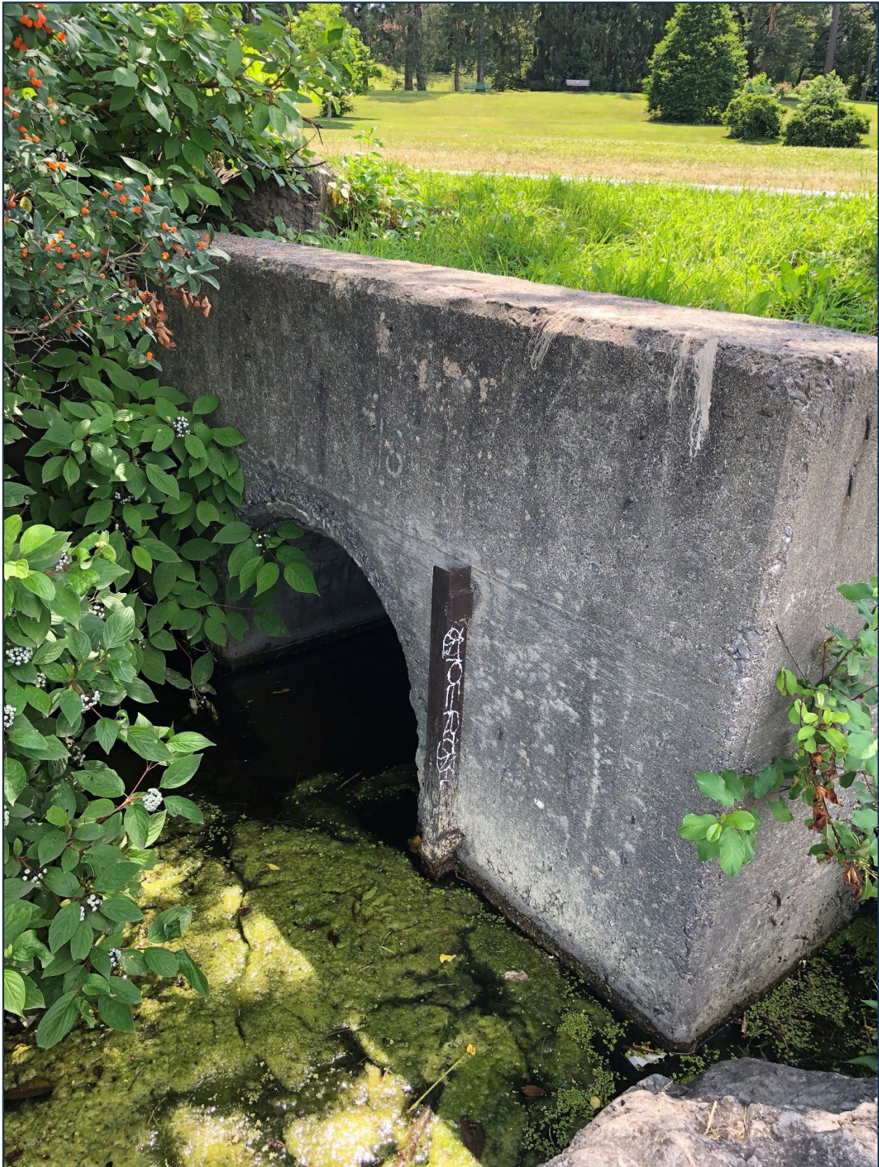
Figure 3-4: Dow's Lake Outfall - July 2022
