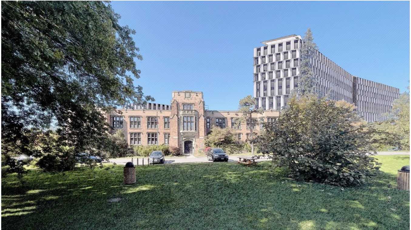
View 11: Saunders Building from front lawn
