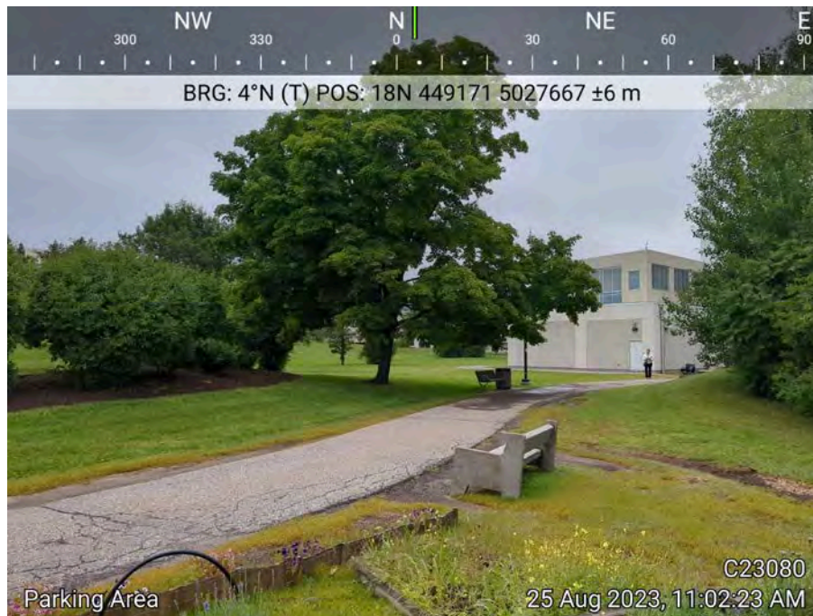
Photo 4: View of existing walking trail, electrical vault in background.
