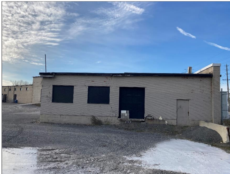
Photo 8 – Property located southwest of the Phase One Property.
