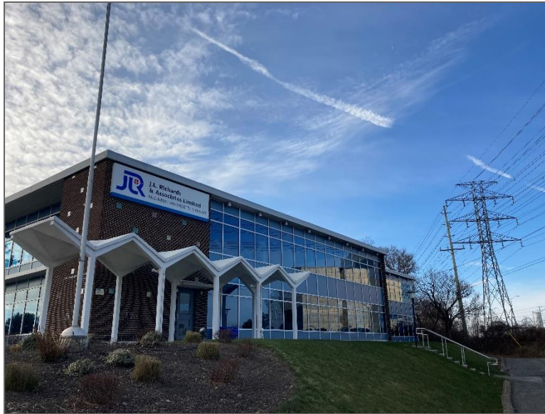
Photo 1 – Site Building (northwest elevation).
