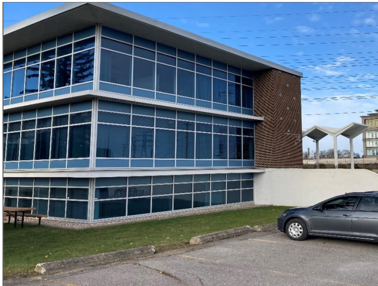
Photo 2 – Site Building (northeast elevation).
