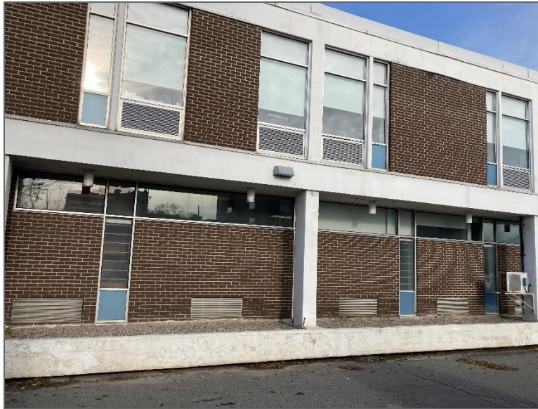
Photo 3 – Site Building (southeast elevation).
