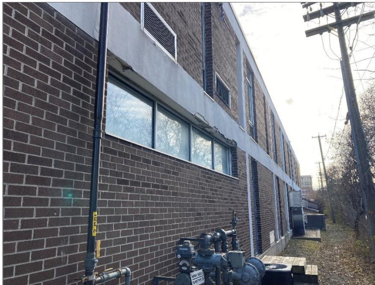
Photo 4 – Site Building (southwest elevation).
