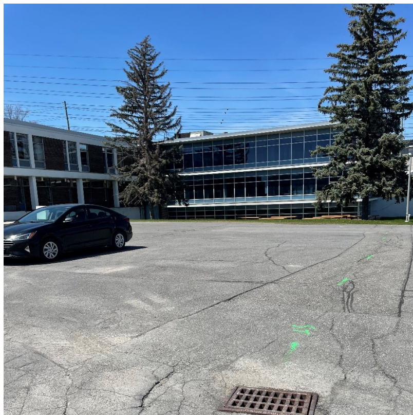
Photo 4: Storm sewer catch basin
