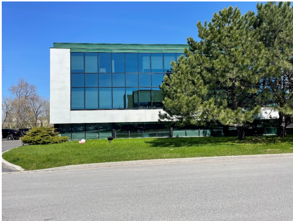
Photo 246: 881 Lady Ellen Place - Former commercial printing location
