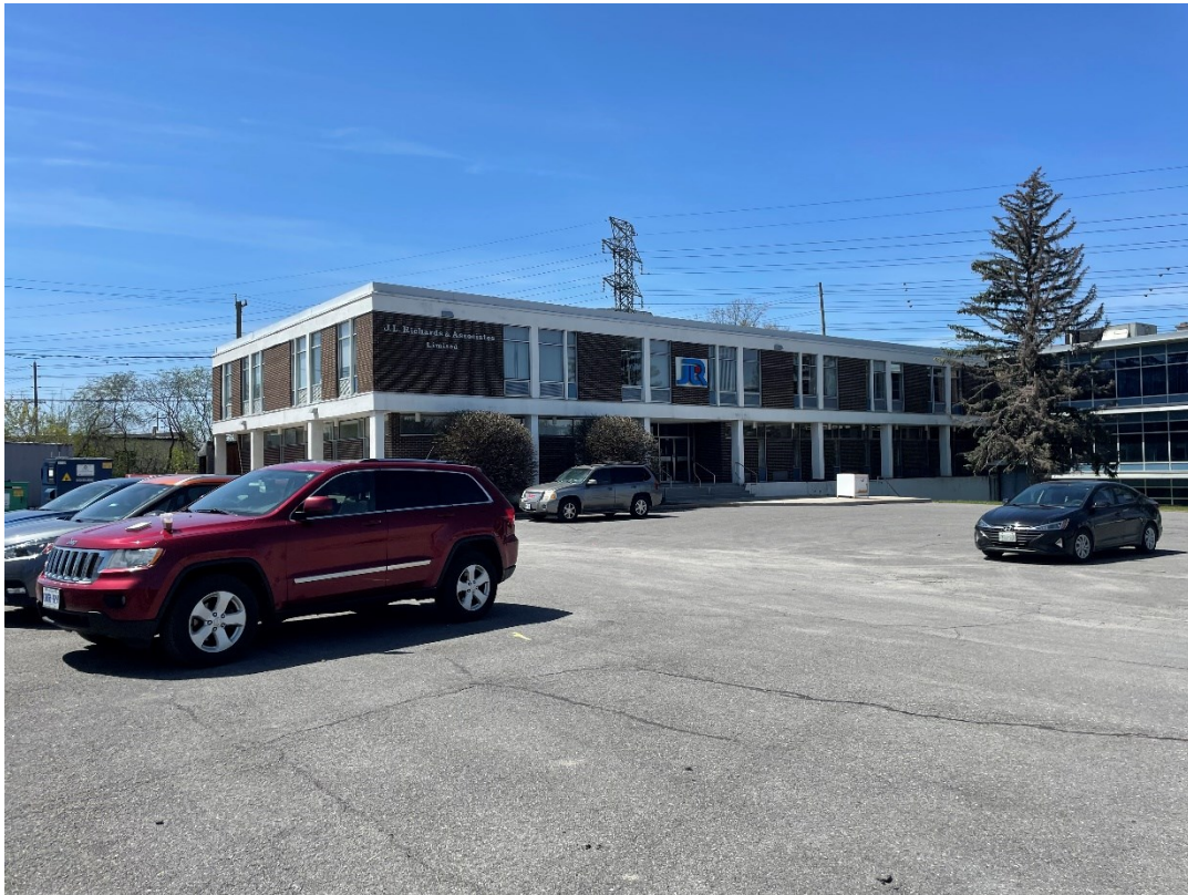
Photo 1: View of building from North
