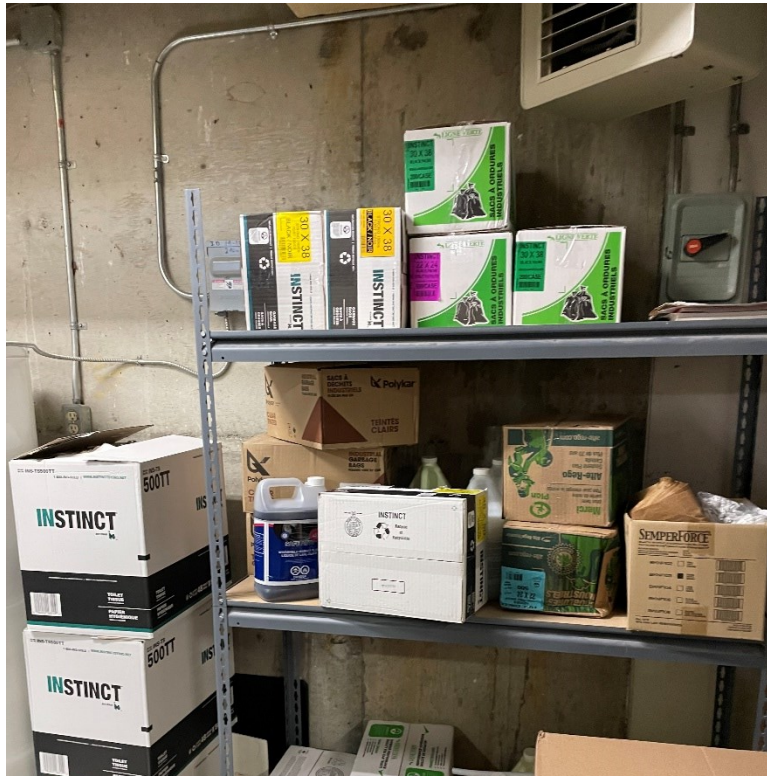
Photo 115: Cleaning supplies in air handler room
