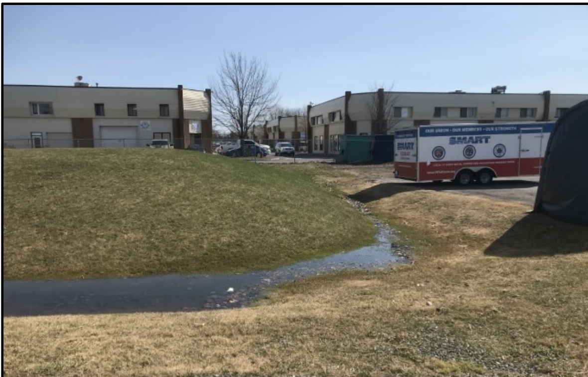
Photo 6: East-facing view of the drainage ditch and surrounding commercial properties.
