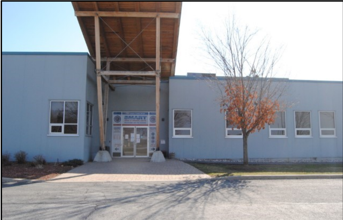
Photo 1: East facing view of the Site building entrance (765 Green Creek Drive)
