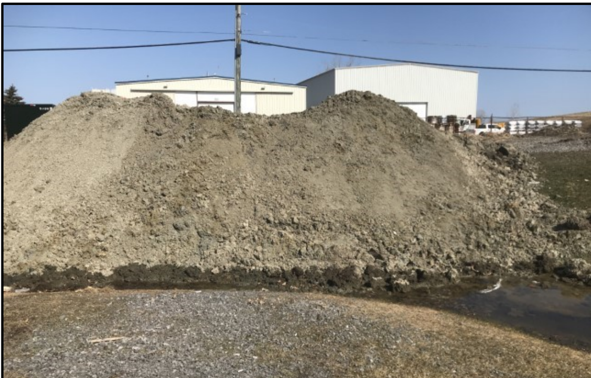
Photo 22: Photo of silty clay native material, originating from the property directly to the north of the Site, excavated during the installation of the onsite transformer.
