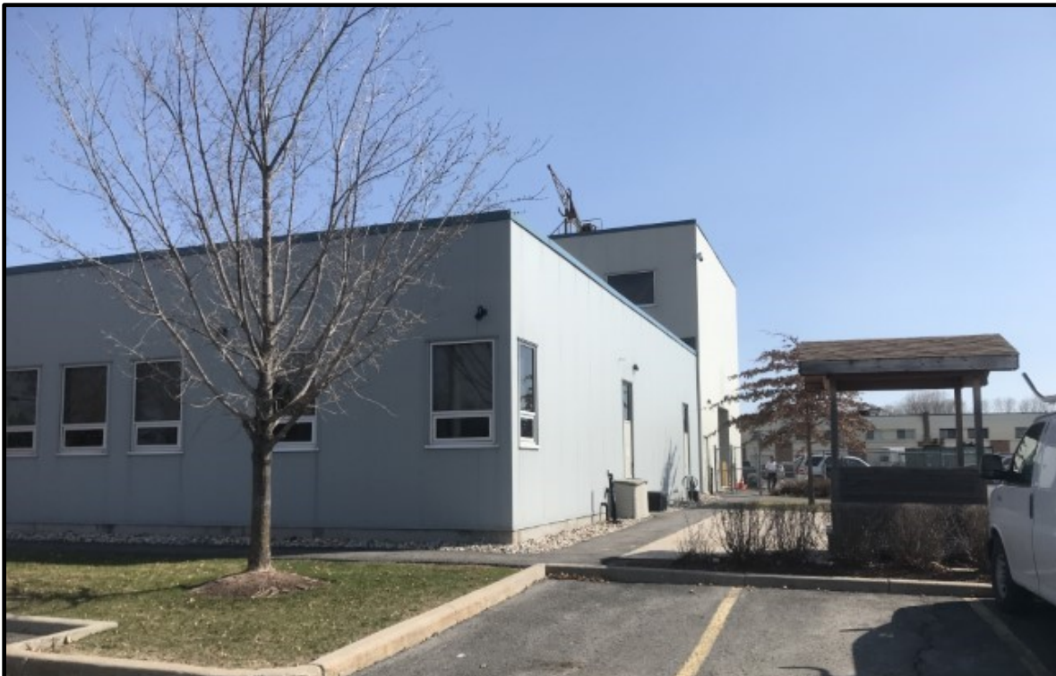
Photo 2: North facing view of the Site building.
