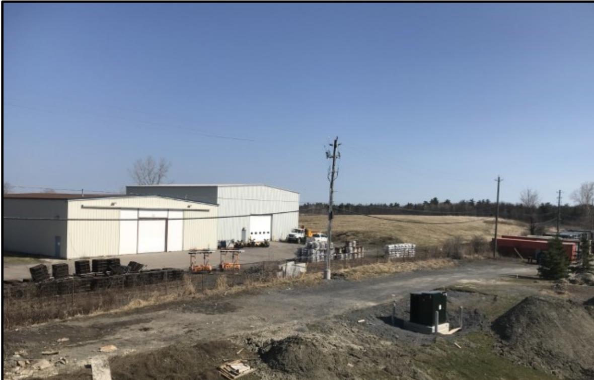
Photo 3: North-east facing rooftop view indicating presence of small fill piles, pad-mounted transformer, drainage ditch, adjacent industrial property to the north (800 Green Creek Drive) and vacant land to the northeast.
