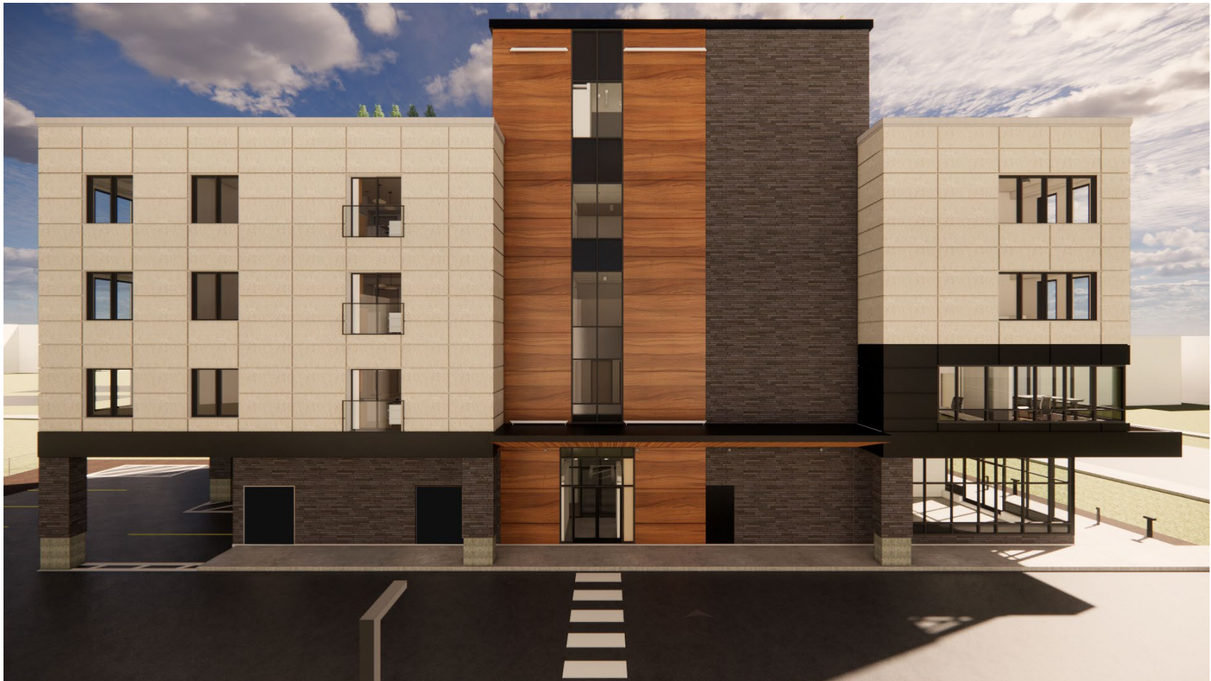
Figure 8- West facade at main residential entrance
