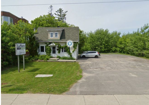
Photo 1: Existing structure at 2663 Innes Road
