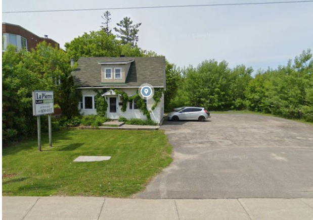
Photo 1: Existing structure at 2663 Innes Road
