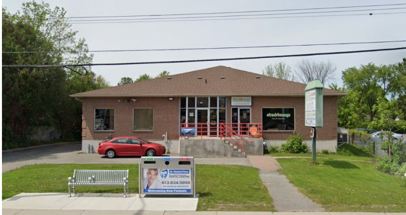
Photo 14: Commercial Multi-Office space abutting Innes Road
