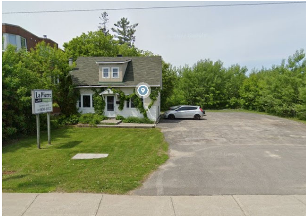
Photo 1: Existing structure at 2663 Innes Road
