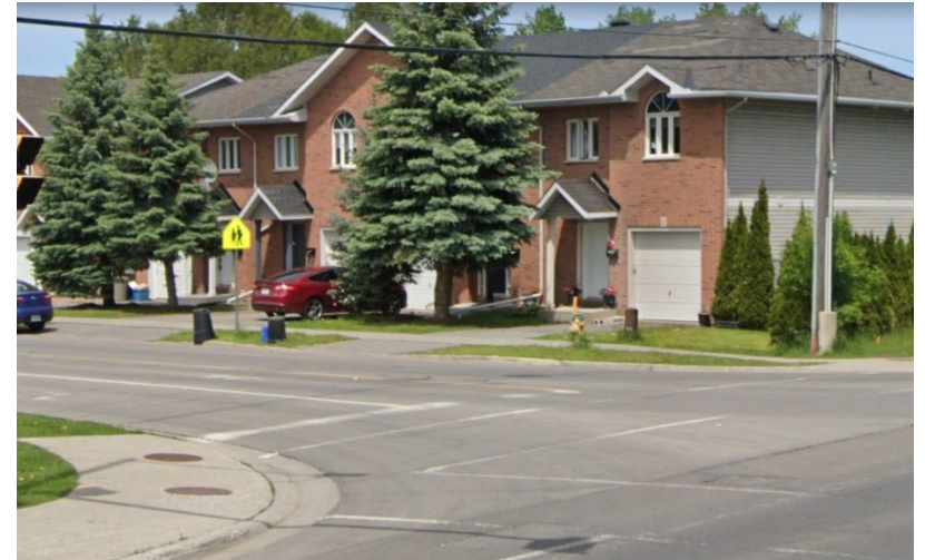
Photo 11: Residential Development abutting Innes Road
