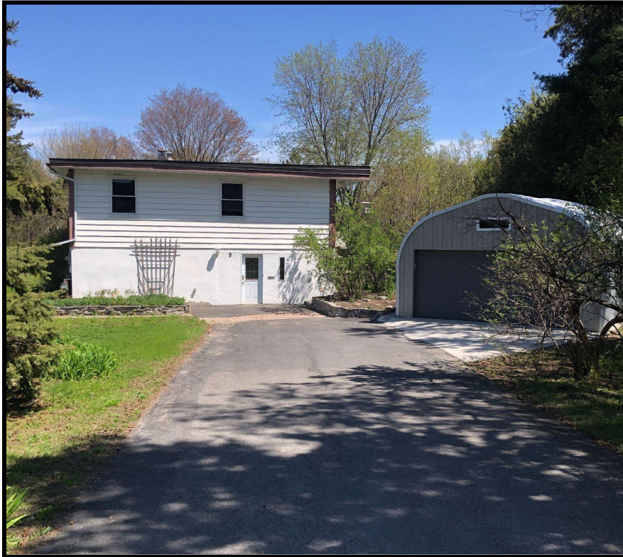
Existing dwelling at 9 Beckenham Ln. looking east.
