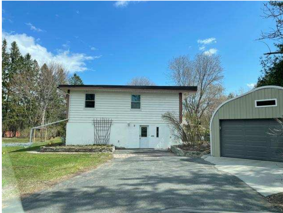
Photograph 3: View of the western portion of the 9 Beckenham Lane property.
