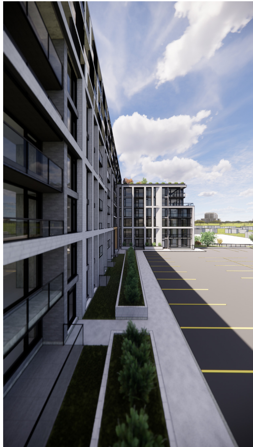
View of Apartment Building and Podium Planters
