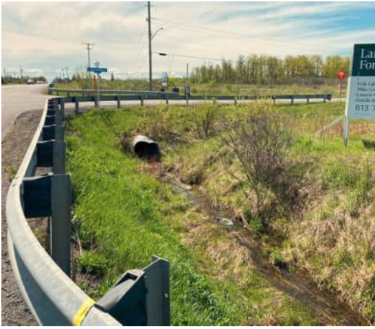
PICTURE 1: Carp Road Ditch @ Russ Bradley Road - Facing South
