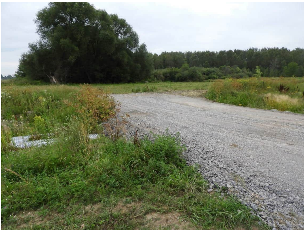
Photo 5: Constructed entrance with twin culverts from Russ Bradley Road over the realigned tributary of Carp River in the west end of the Forb Meadow. 11 August 2021.
