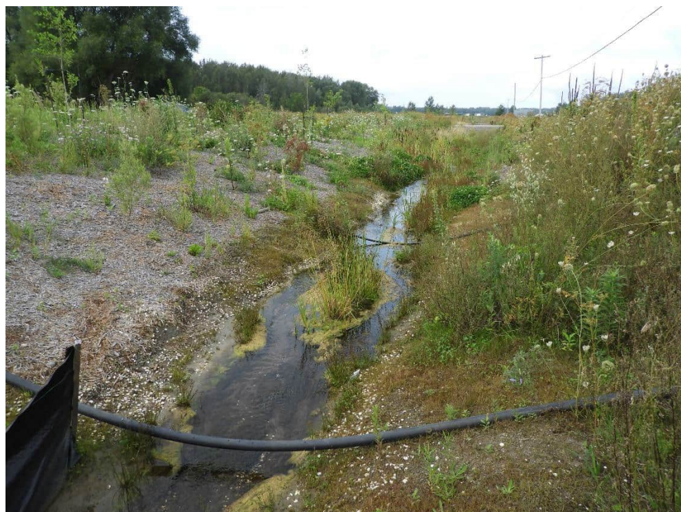
Photo 4: Upstream view of the tributary of Carp River (looking southwest) which was realigned parallel to the south side of Russ Bradley Road (to the right of the photo). 11 August 2021.
