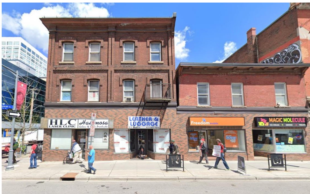
Figure 12: A view of 211 Bank Street with the two-storey unit.
