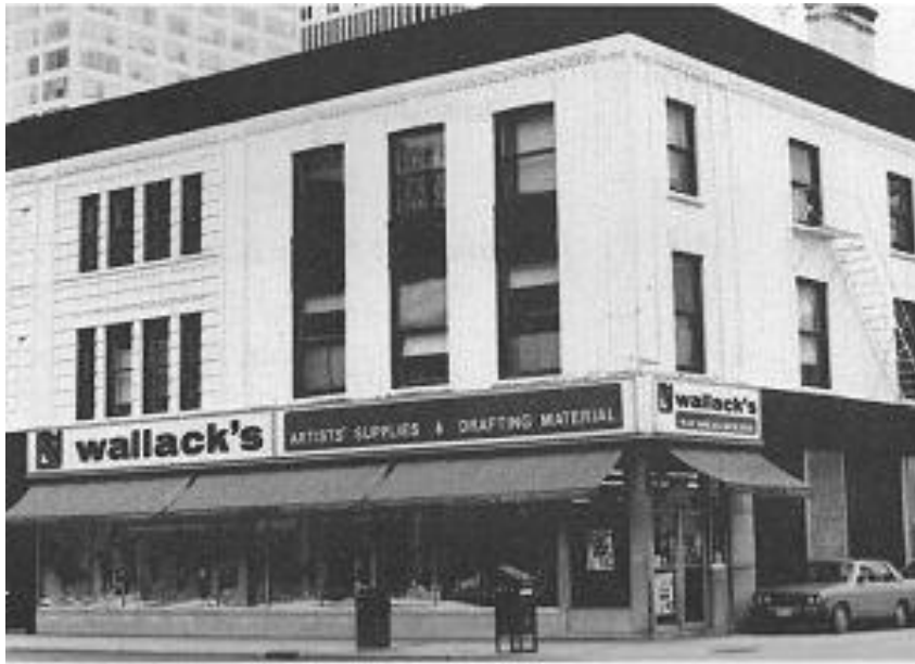
Figure 19: A view of 231 with the retail entrance shifted from its original central location to the corner and the upper façade painted white.
