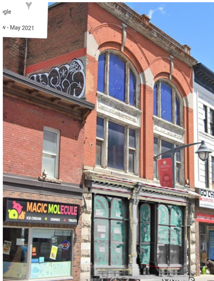
Figure 23: Examples of comparable historic Ottawa shopfronts used as models to guide restoration of 119 Bank Street.
