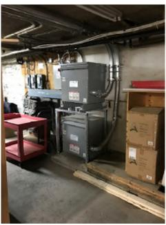
**Photograph No. 10** View of the air cooled transformers in the basement.
