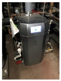
**Photograph No. 9** Example of a natural gas fired boiler in the basement.
