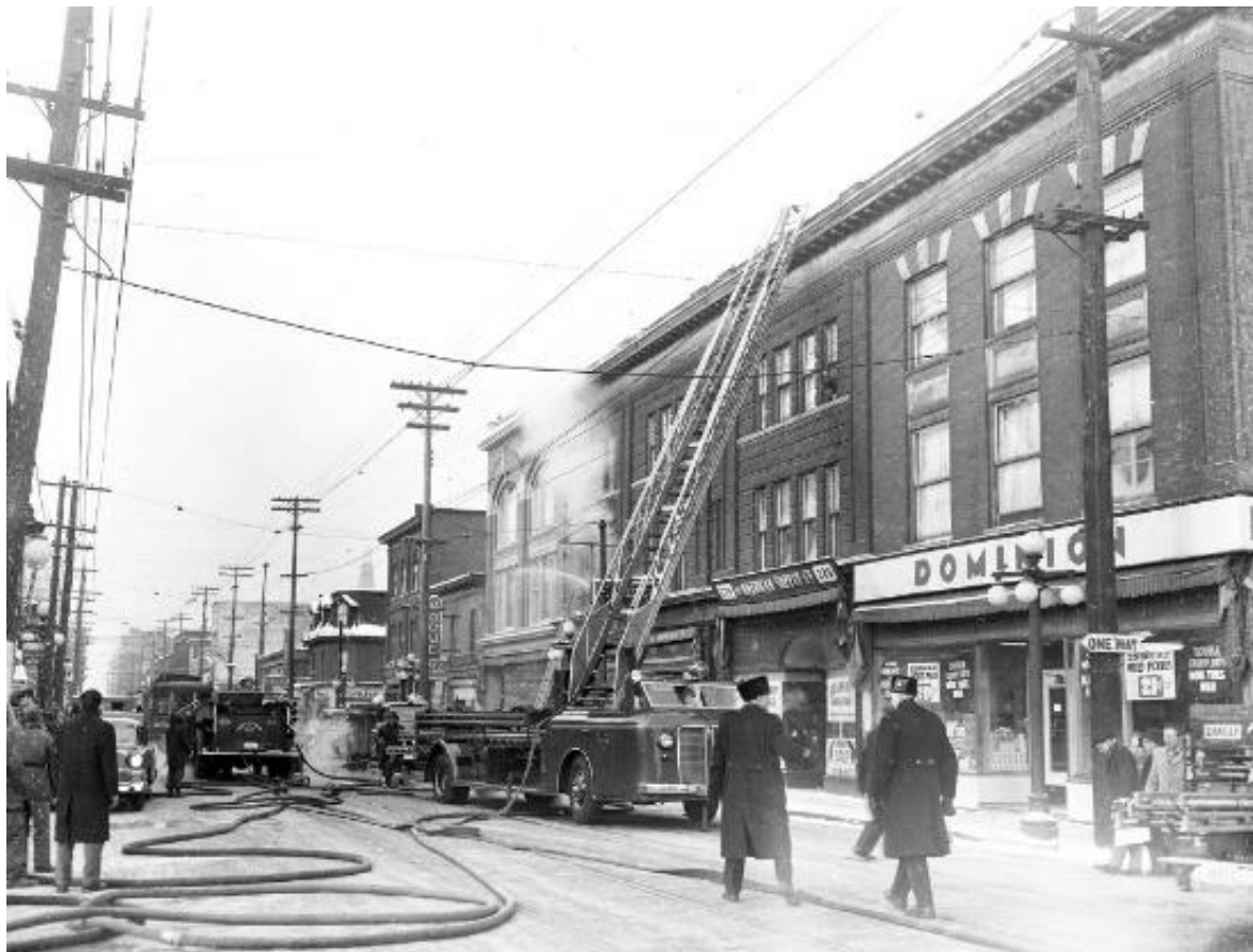
Figure 1: Bank Street view, c.1950. Source: City of Ottawa Archive.
