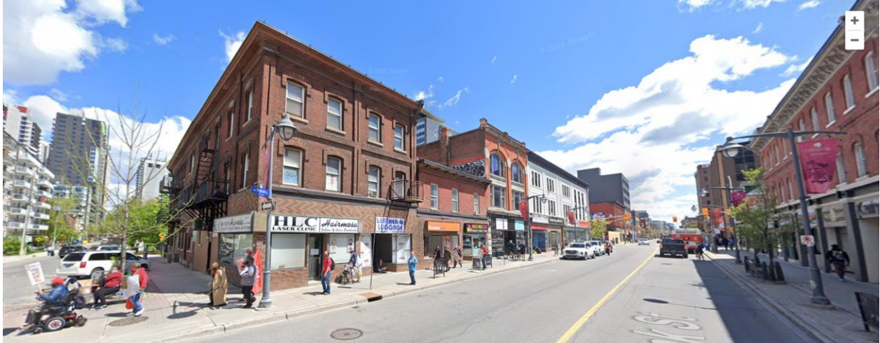
Figure 7: Street view of the properties looking south-east.
