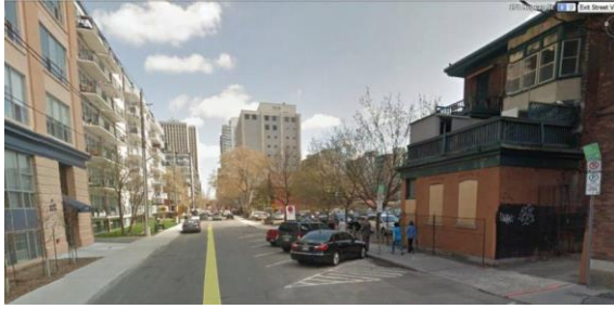
Figure 4: View looking east on Nepean St. from Bank St. The building to the right is part of the Richcraft's development and has been demolished. On the left is the Acart Building, a 6-storey residential development. Source: Google Earth
