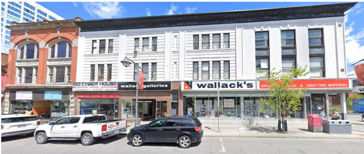
Figure 14: The painted brick commercial range 223-231 occupies the southern half of the block with the Wallacks Art Supply wrapping around the corner and extending along Lisgar Street.
