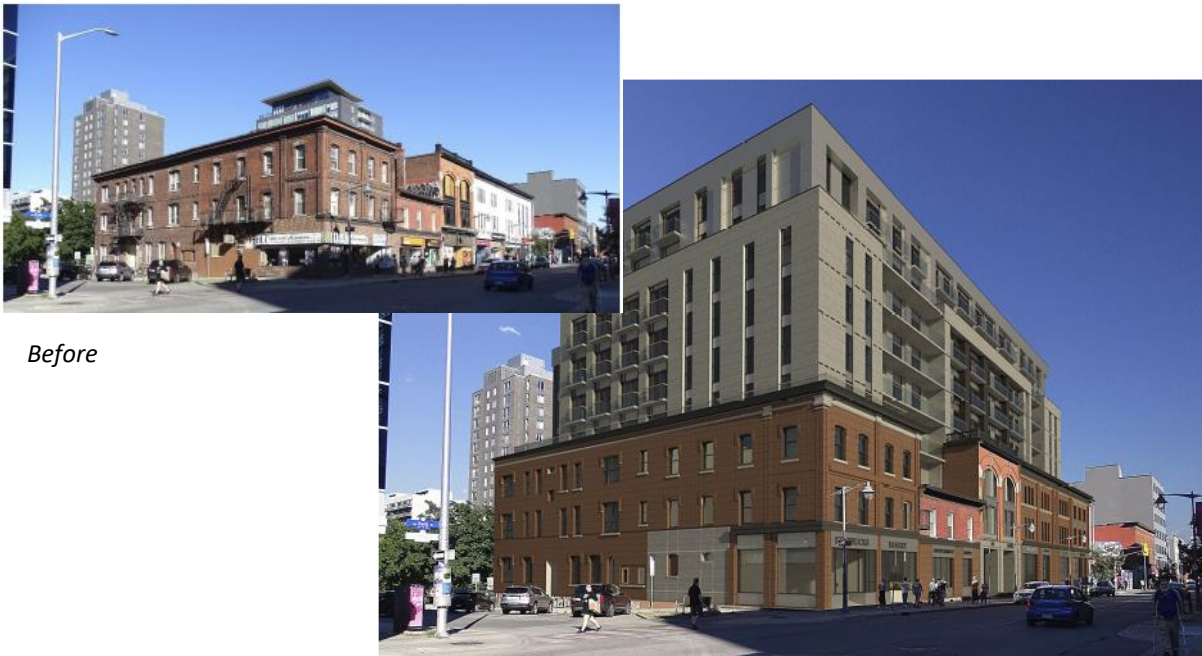
Figure 22: View of the development site looking south-east showing the existing buildings and the new 9-storey development. Source: Woodman Architecture 2023
