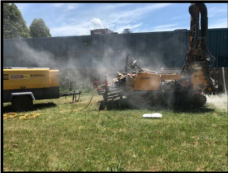
Drilling at MW2 – June 19, 2020
