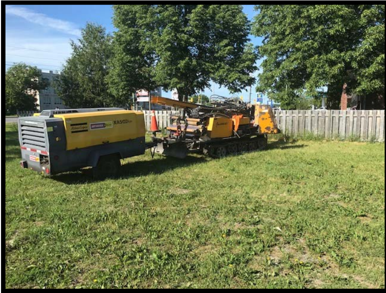
Drill Setting Up at MW1 – June 19, 2020
