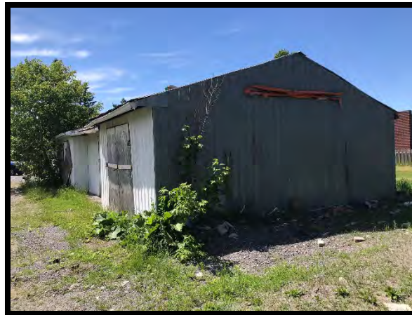
The Site (Shed, north-facing rear)
