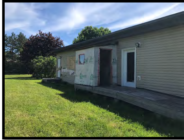
The Site (Commercial trailer – north-facing rear)
