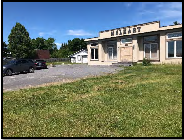
The Site (Commercial trailer – south-facing front)
