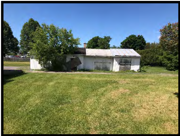
The Site (Shed, east-facing side)
