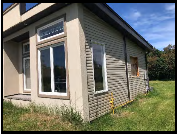
The Site (Commercial trailer – east-facing side)
