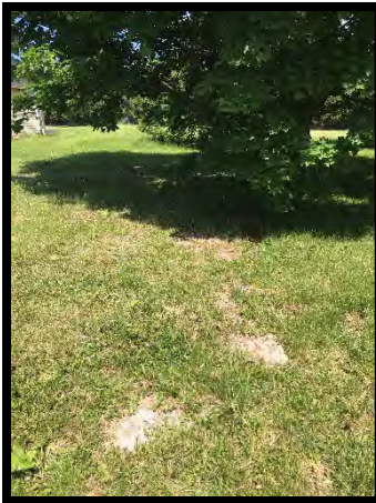
The Site (Buried concrete, front-eastern portion of site)
