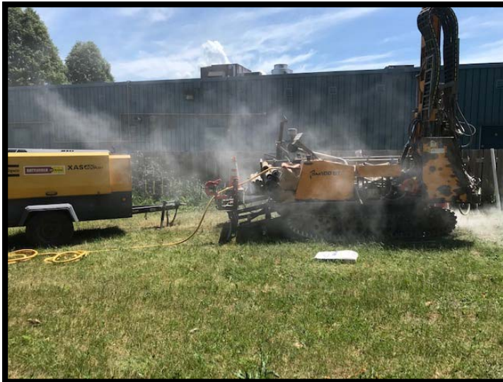
Drilling at MW2 – June 19, 2020
