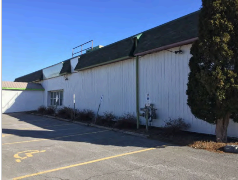
Photo 3 – Site Building B (west elevation).
