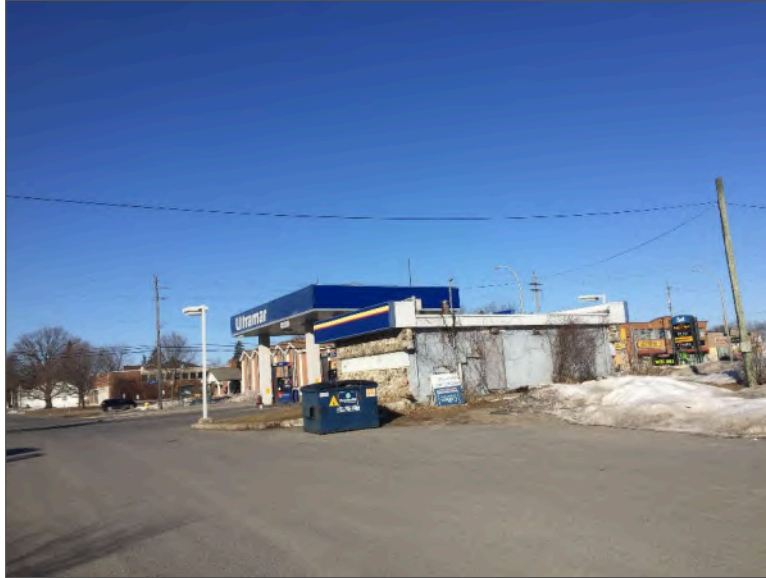
Photo 7 – RFO located west of the Site.
