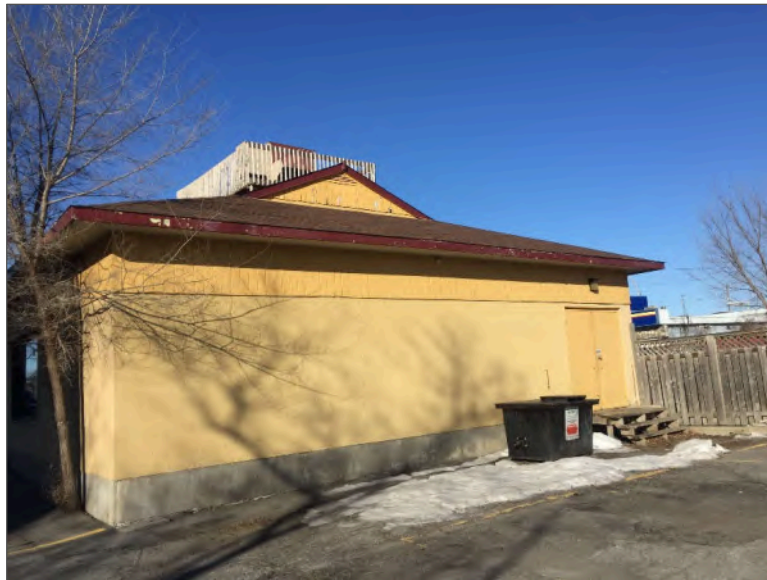
Photo 2 – Site Building A (northeast elevation).
