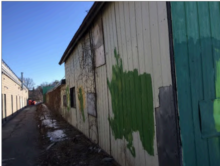
Photo 4 – Site Building (north elevation).
