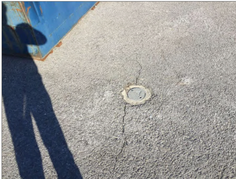
Photo 8 – Groundwater monitoring well on the northwest portion of the Site.
