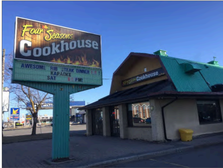
Photo 1 – Site Building (southeast elevation).
