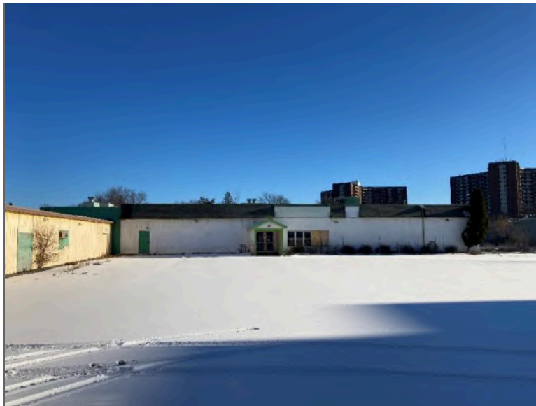
Photo 4 – Site Building B (west elevation).
