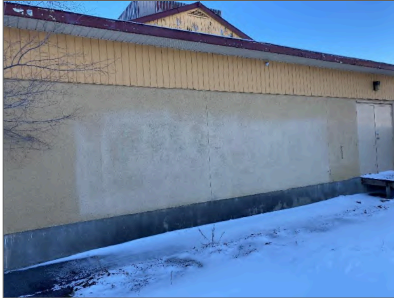
Photo 3 – Site Building A (east elevation).
