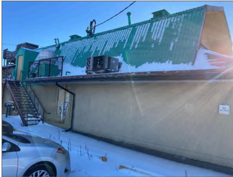
Photo 1 – Site Building A (north elevation).
