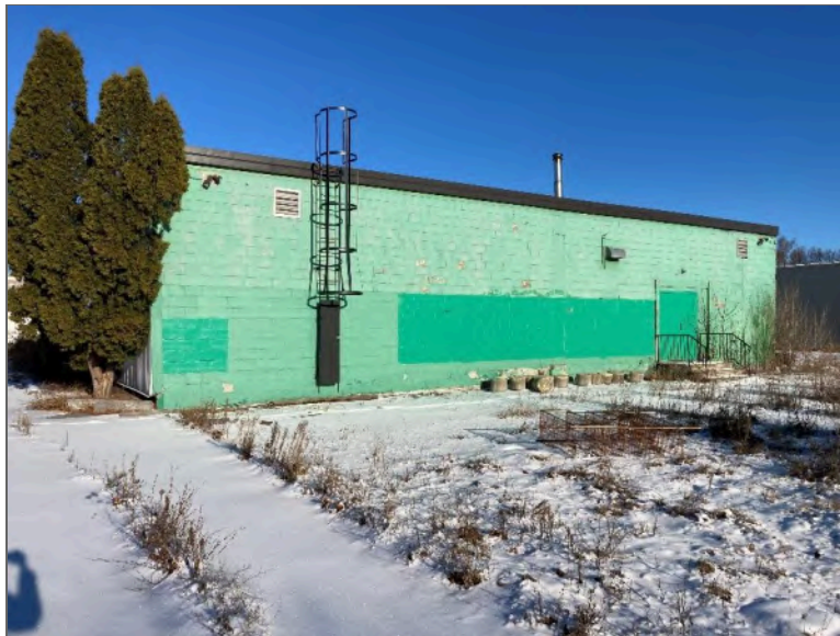
Photo 2 – Site Building B (south elevation).
