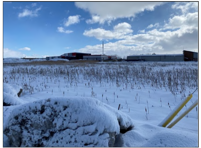
2. 5210 Innes Road – View of the Site looking southeast.
