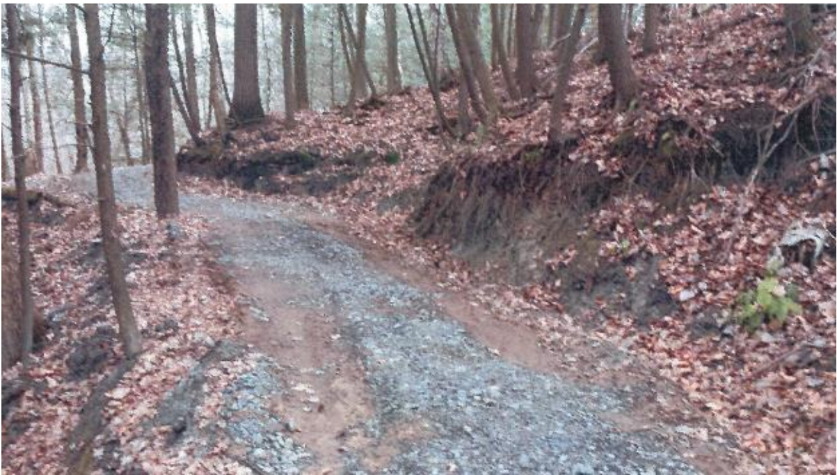
Photo No. 6 – Erosion of cut uphill of pathway. Cut approximately 16 m long x 0.5 m to 1 m high.
