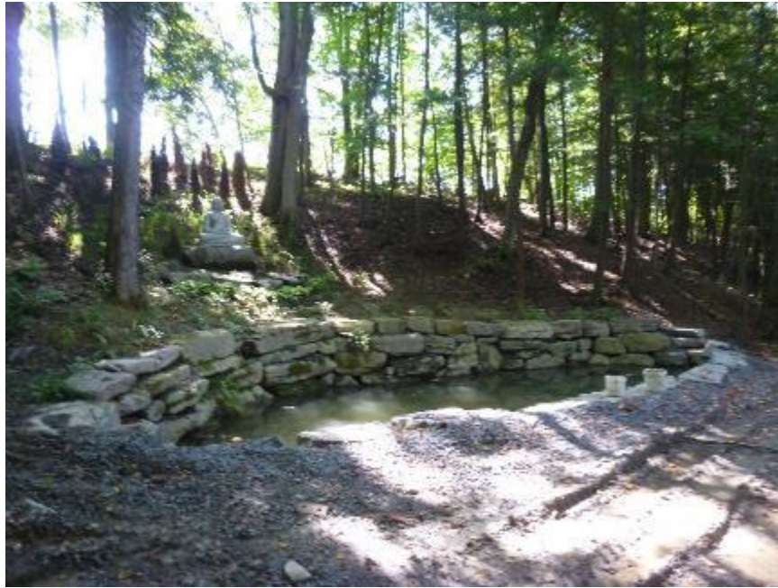
Photo No. 26 –Retaining wall at pond location.
