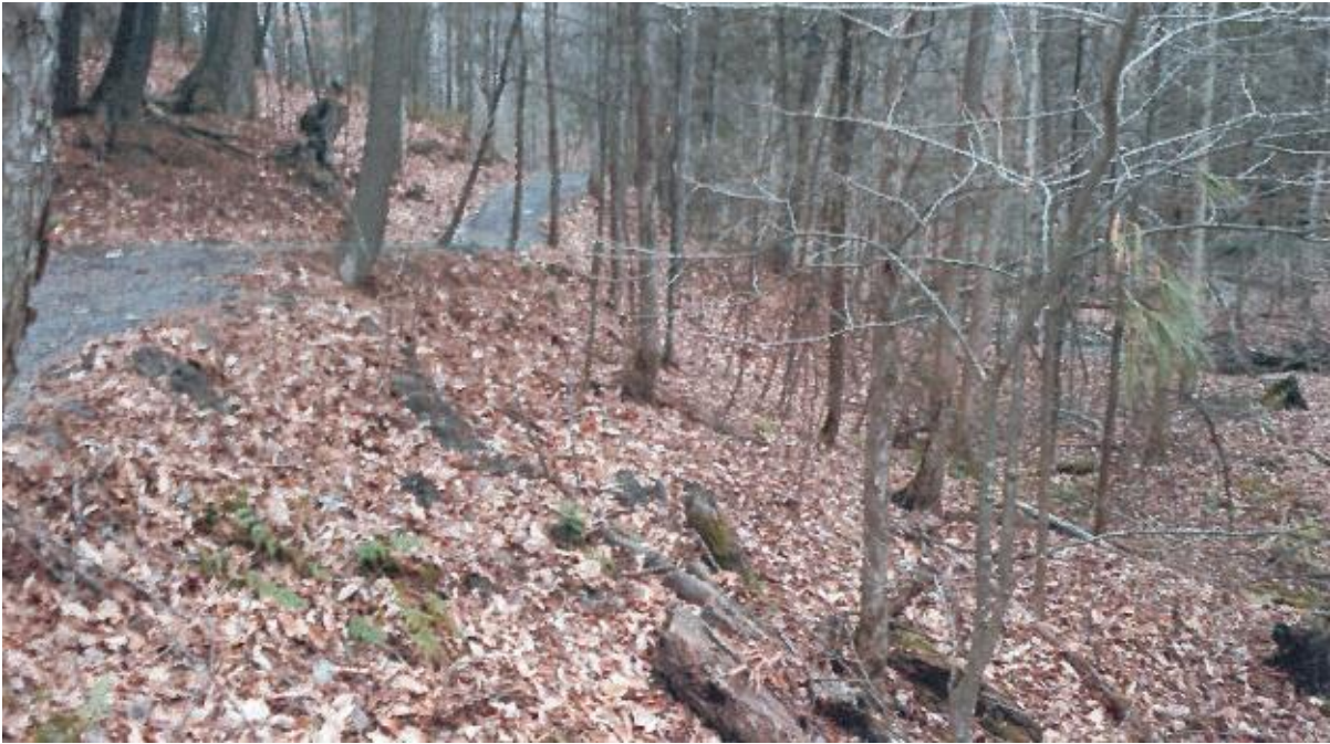
Photo No. 22 – Erosion below pathway. Cut approximately 30 m long x 0.5 to 2 m high.
