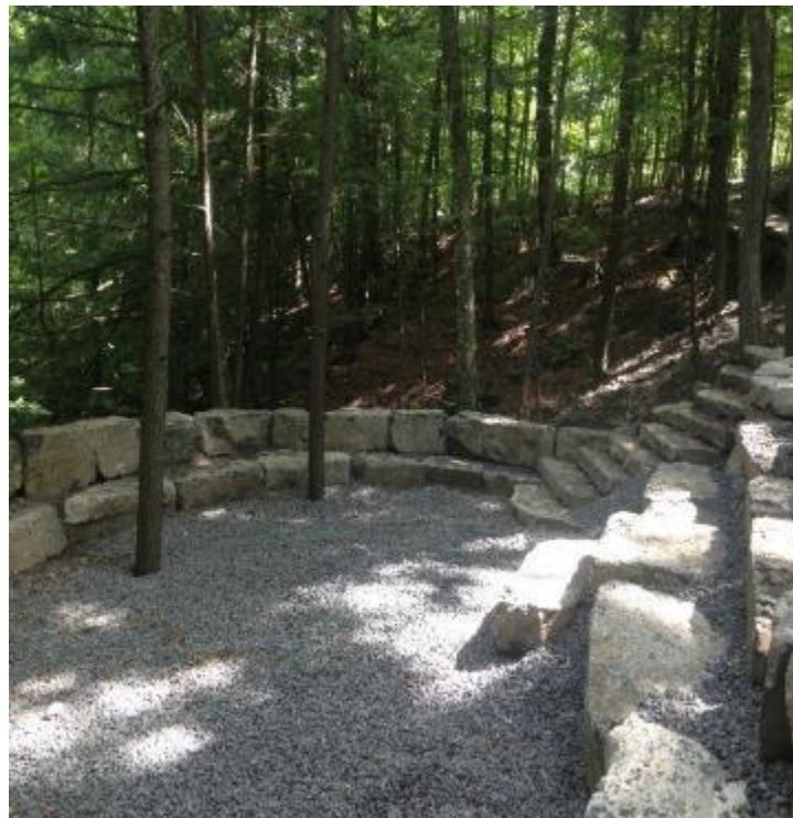
Photo No. 27 –Retaining walls across from the pond and the pathway.
