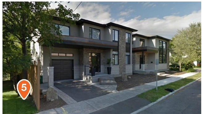
Figure 9: Looking northeast on Gould Street
