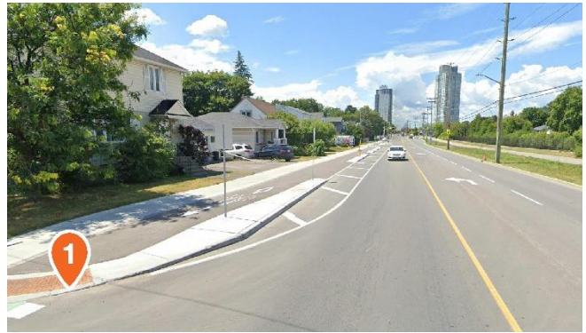
Figure 5: Looking west along Scott Street
