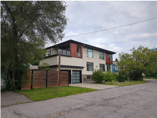
53 Gould Street, viewed from Rockhurst Road
