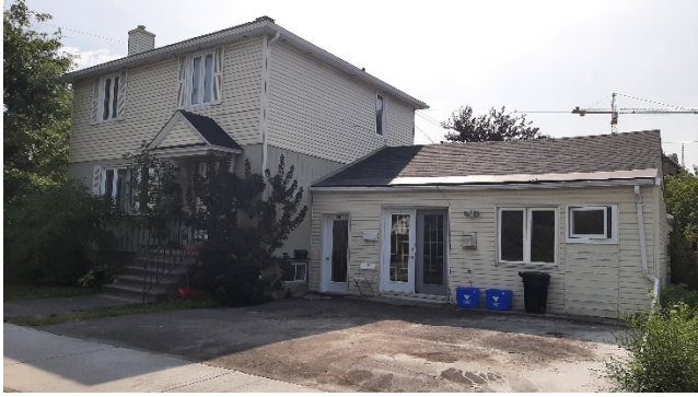
1806 Scott Street, viewed from Scott Street ★
