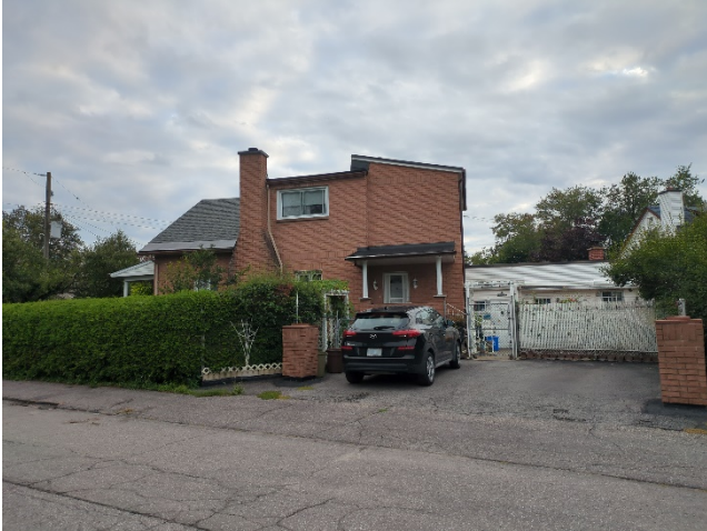
323 Oakdale Avenue, viewed from Rockhurst Road
