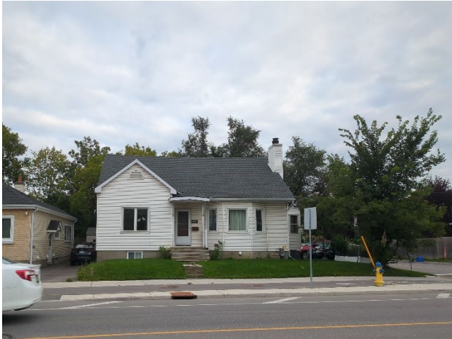
1798 Scott Street, viewed from Scott Street
