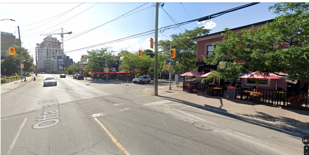
Image 1.1.5. (This area is outside of the study area shown on the context map) – looking west from Richmond Rd. near intersection of Western Ave. showing the vibrant main street, within walking distance of the proposed site. Shopping, services, and employment opportunities for tenants are easily accessible.
