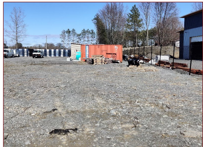
Photograph 4 – Fill material present on the southwest portion of the Site.
