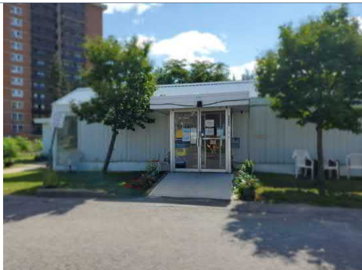
Picture 1 – Site building on RSC Property (facing south)
