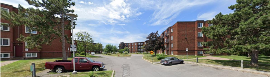
Figure 15. Surrounding Built Form: Mid-rise Residential Buildings West of the Site at 2041 and 2044 Arrowsmith Drive (Looking West)
