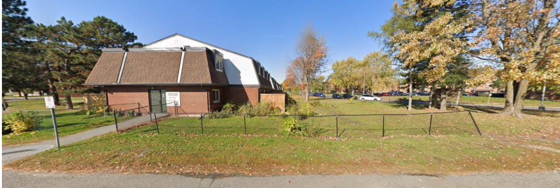
Figure 13. Surrounding Built Form: Low-rise Residential North of the Site at 1958 Jasmine Crescent (Looking Northwest)
