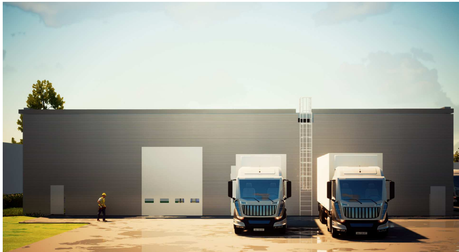
3 - REAR VIEW OF SITE
