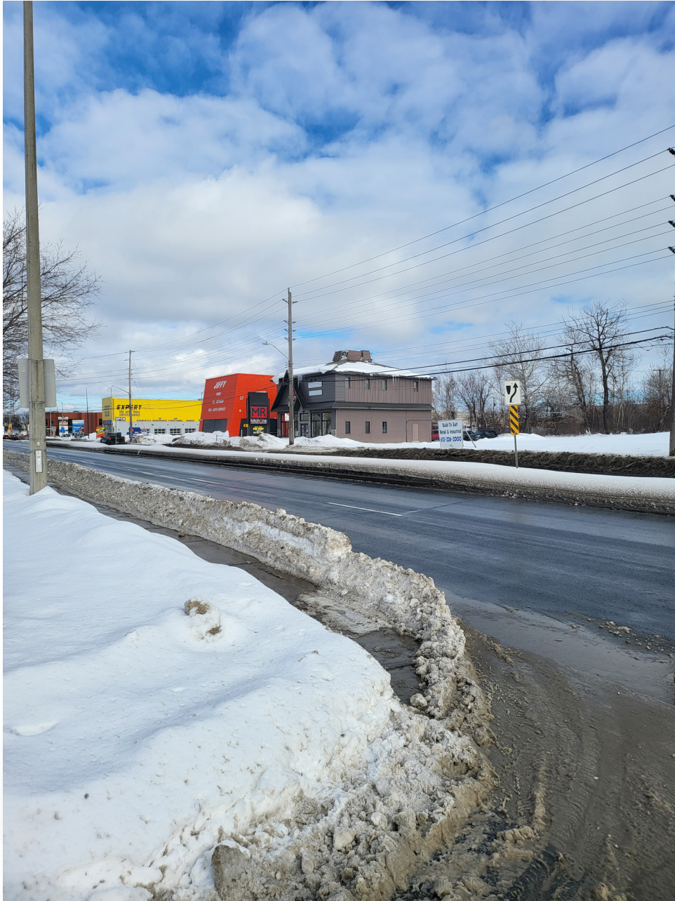
Merivale Frontage Looking North
