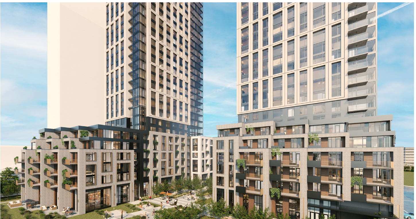
Figure 17.0 - View looking North-West, West building podium terraces.
