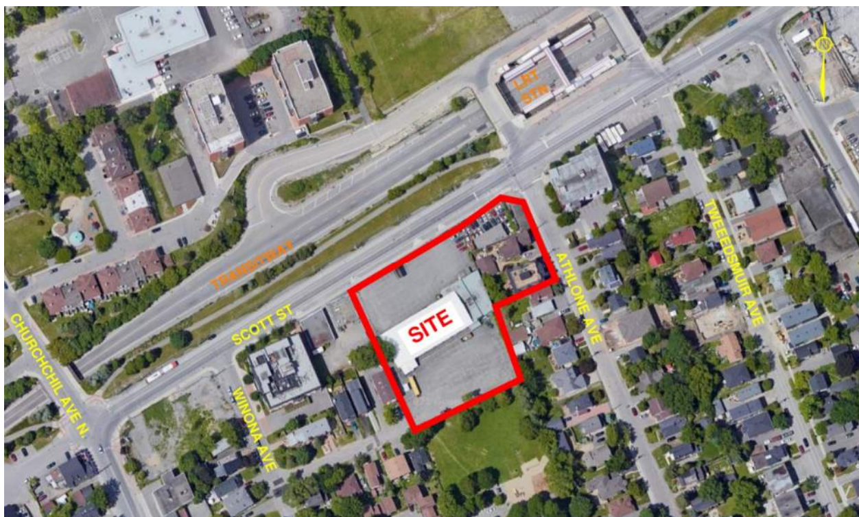
Figure 1: Aerial View of the Subject Site
