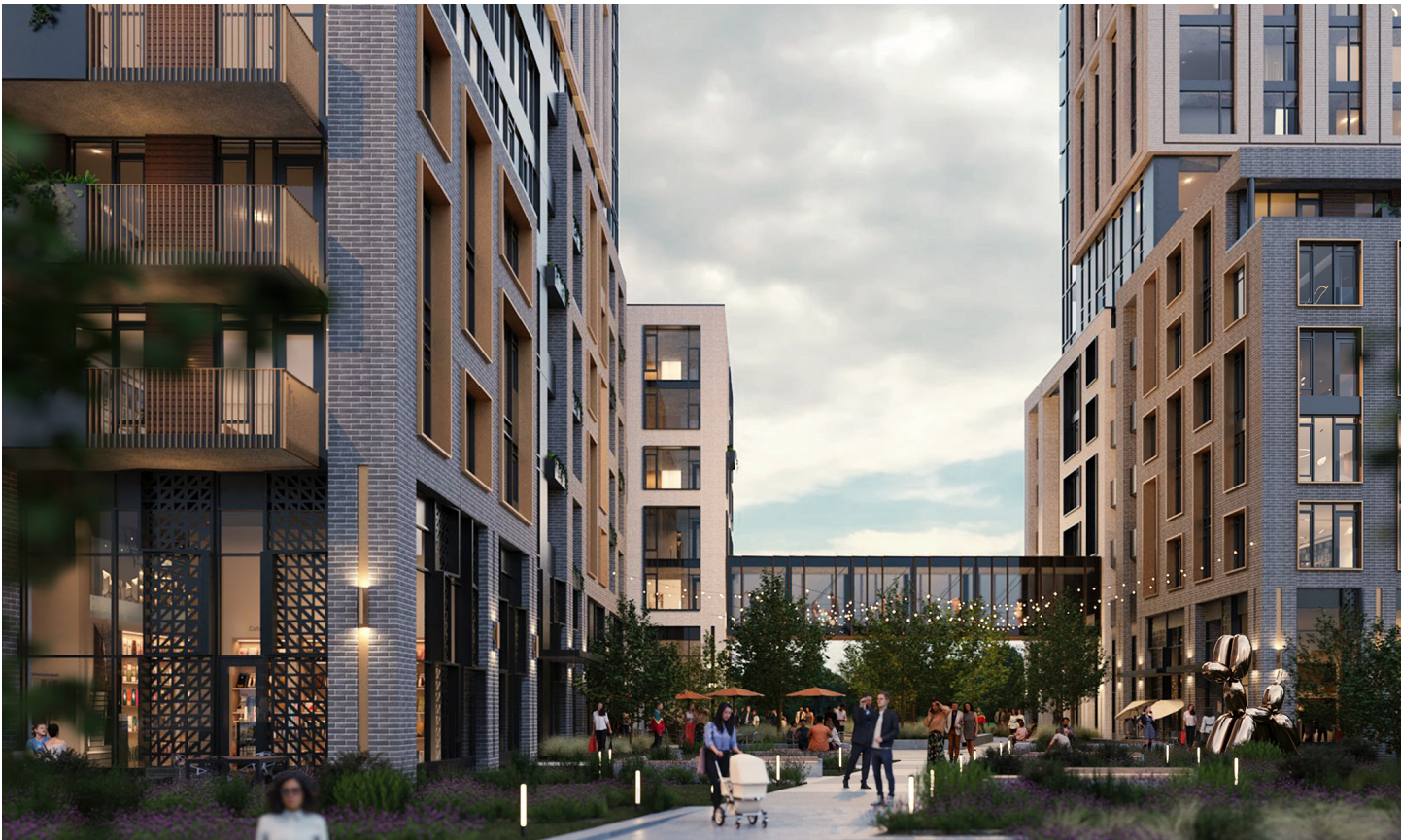
Figure 14.0 - View of the pedestrian plaza linking Scott Street and Lion's Park.
