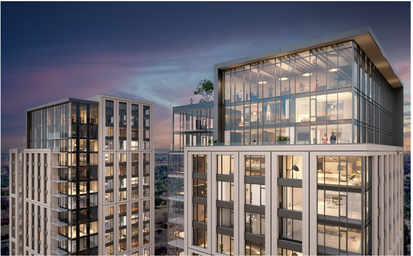
Figure 21.0 - View of tower crowns looking South-East.
