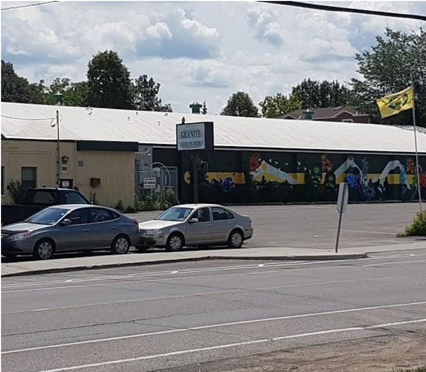
Figure 3.0 - Existing Granite Curling Club, 2026 Scott Street.
