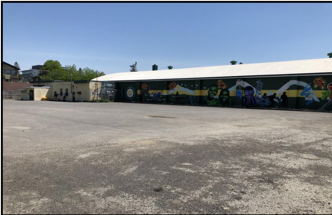
Photograph 4: View of the curling arena at 2026 Scott Street, facing southeast from Scott Street.
