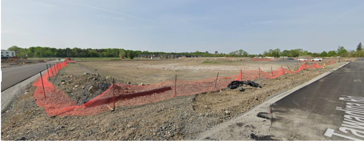
Figure 3: View from intersection of Tawadina Road and Michael Stoqua Street -- Looking south-west into site
