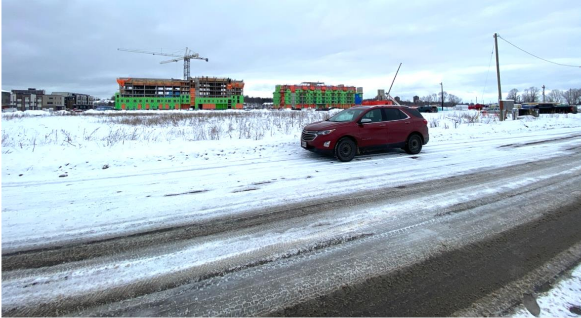
Figure 6: View of Site Looking South. Development South of Hemlock Under Construction In Background
