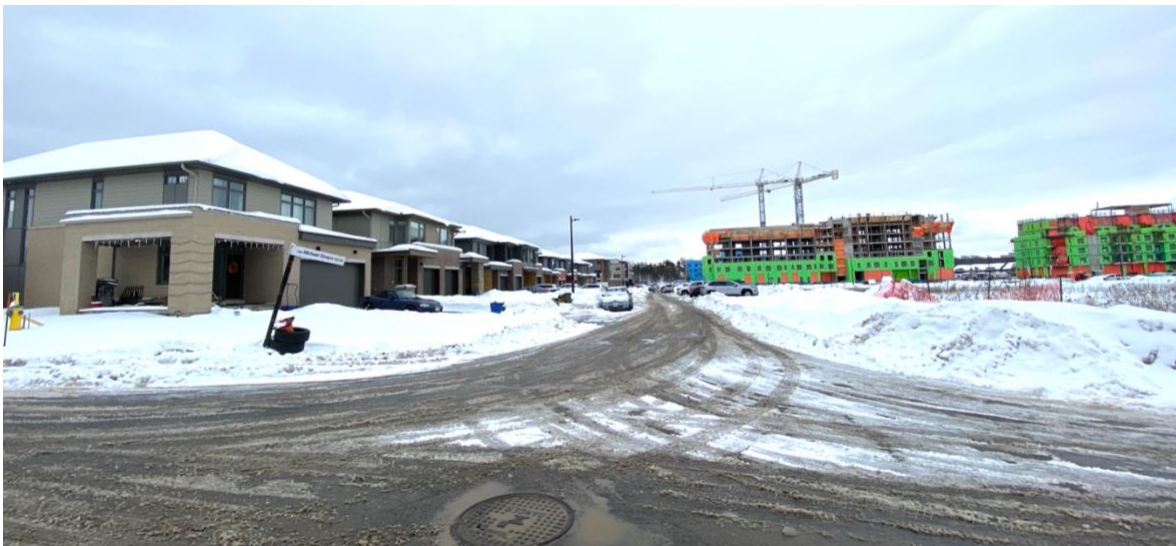
Figure 7: View Looking South on Michael Stoqua. Site on Right.
