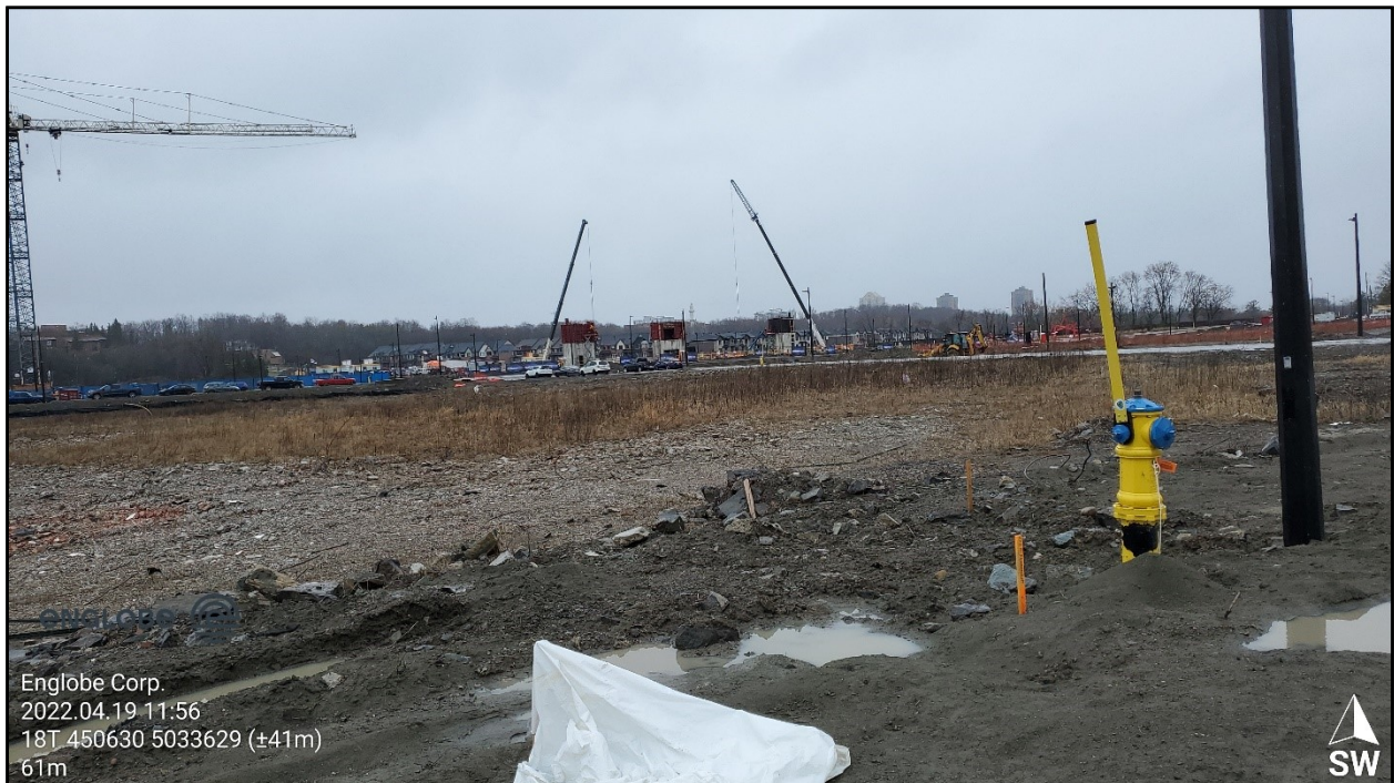
Photograph 2: View of Block 11 Parcel 1 facing southwest.
