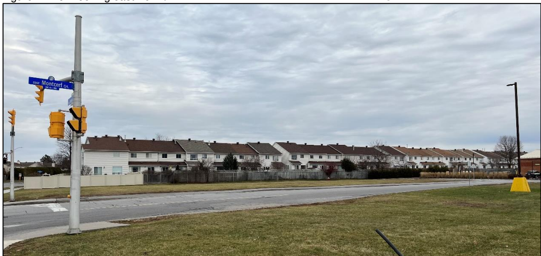
Figure 4: View looking east from Jeanne D'Arc Boulevard South and Montcerf Court.
